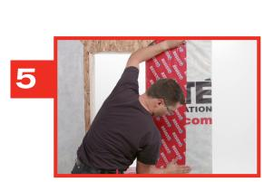
Install a membrane strip from 5 to 7.5 cm (2 to 3 in) on the weather barrier of the joist.
