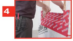
Apply a REDZONE strip on the lower part of the window and cover 5 to 7.5 cm (2 to 3 in) of the weather barrier. Cut the membrane on each side of the opening and adhere it with a membrane roller.
