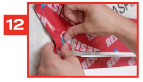
Seal the metal flashing corners by installing a REDZONE membrane strip obliquely on each end.
