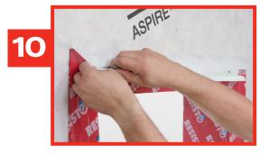
Fold the weather barrier membrane in place. Cut 2.5 cm (1 in) of the weather barrier to clear the metal flashing.
