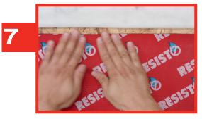
Lift the upper weather barrier. Adhere a REDZONE strip to cover the top of the window.
