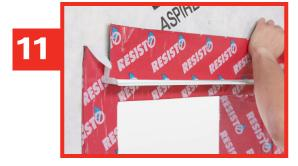
Apply a REDZONE strip to the weather barrier membrane and metal flashing to ensure the continuity of the air barrier.
